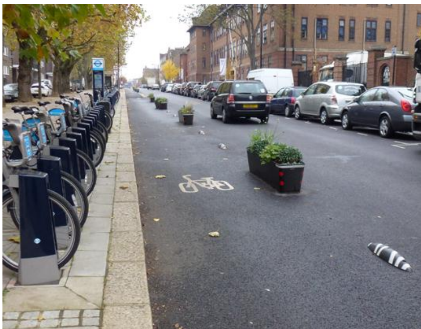
Figure 7: Armadillos and planters provide light segregation in Camden
